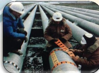
First Service Project: Pipe Marker install on the Alaska Pipeline in 1984.
